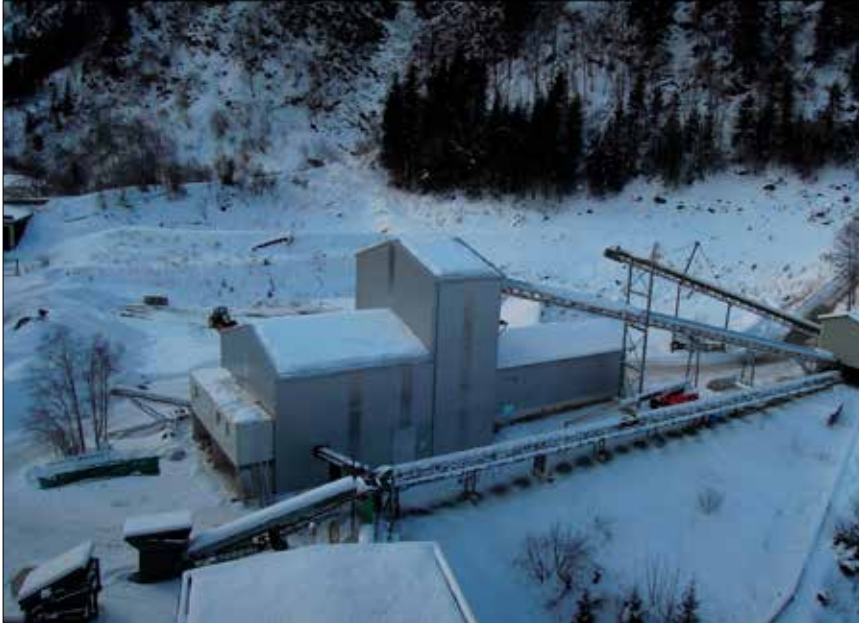
Figure 2. Sorting island installed at the Mittersill tungsten mine in Austria. 1
